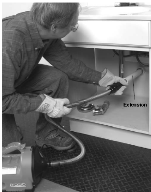
Figure 10 – Example of Extending Drain to Within 6" (15 cm) of AUTOFEED.
