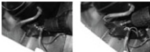
(2) Loosen two screws on comp base
