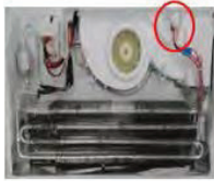
Defrost Heater Defrost Sensor
